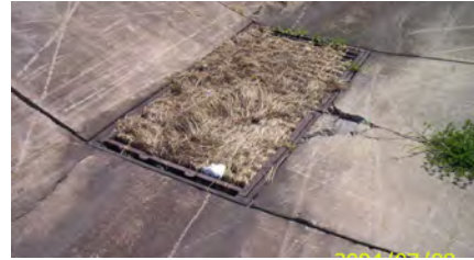
Storm Drain Inlet
